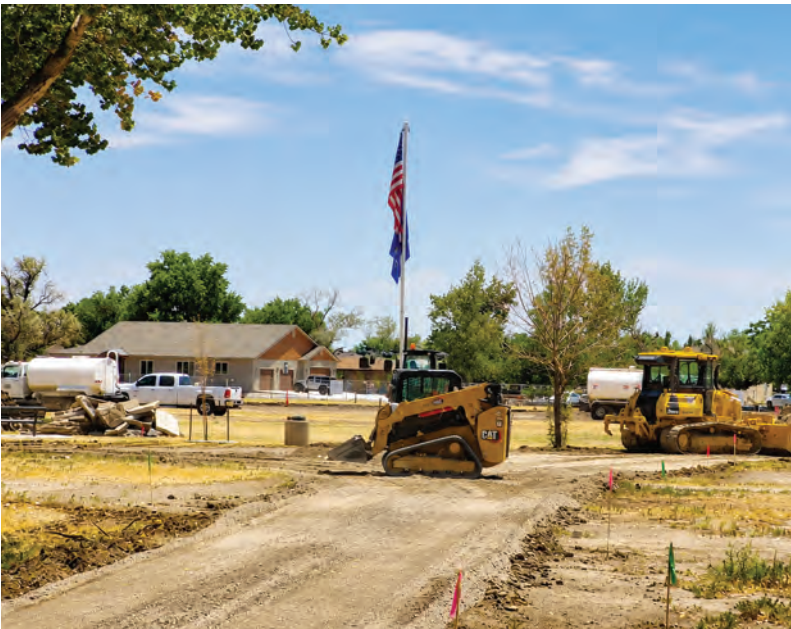
Fencing surrounds Laura Mills Park as construction begins on the city's renovation project. Photo by Lori Kaiser.
