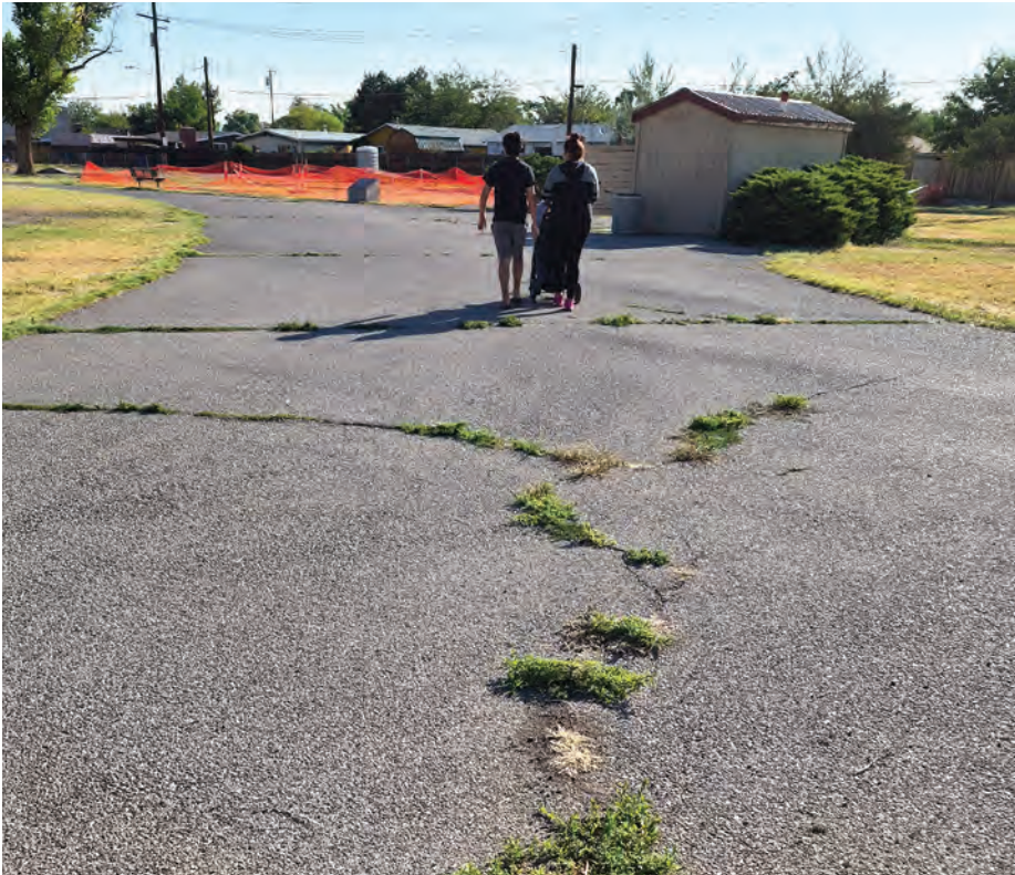
Residents walk through Laura Mills Park as construction begins on a project to replace the park's aging asphalt walking paths with wider, more accessible concrete paths designed to improve drainage and accessibility. Portions of the park will remain open while work continues. Photo by Lori Kaiser.
