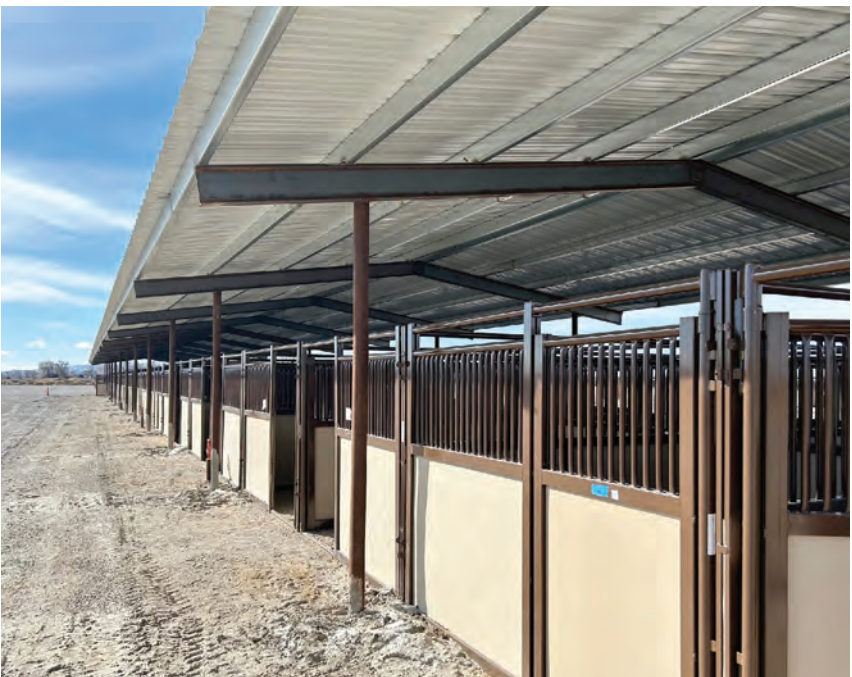
Horse stalls on Miners Road for fire evacuees. Photo courtesy of Churchill County.
