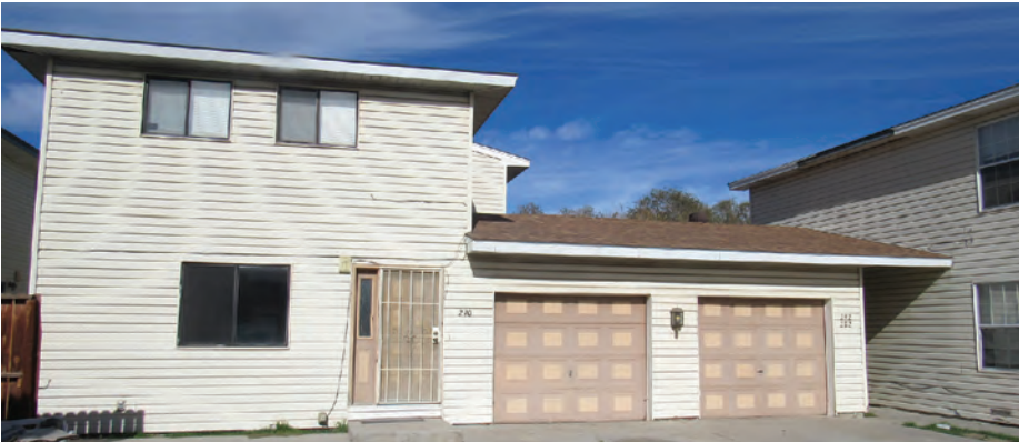
New Pass House and Day Center unit awaiting renovation. Photo by Jim Fleming.
