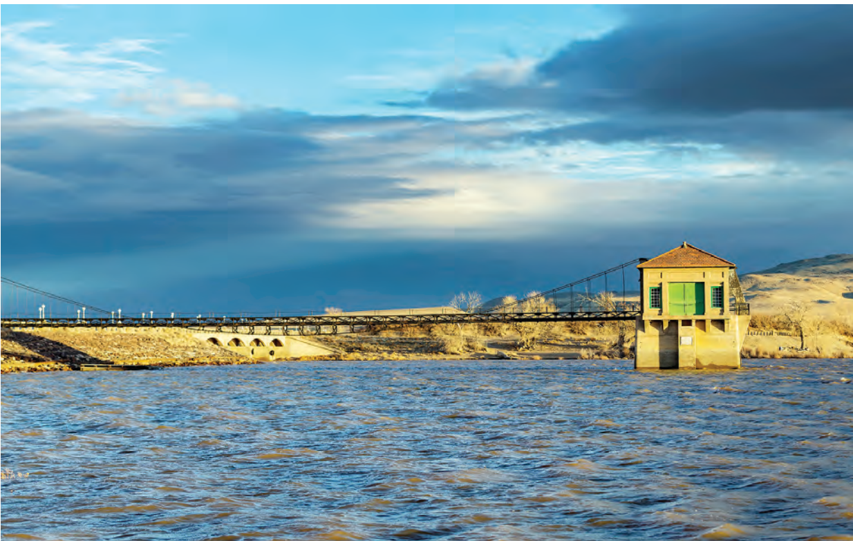
Tower at Lahontan Dam. Gates below feed water to the hydroelectric power plant via a large pipeline. File photo.
