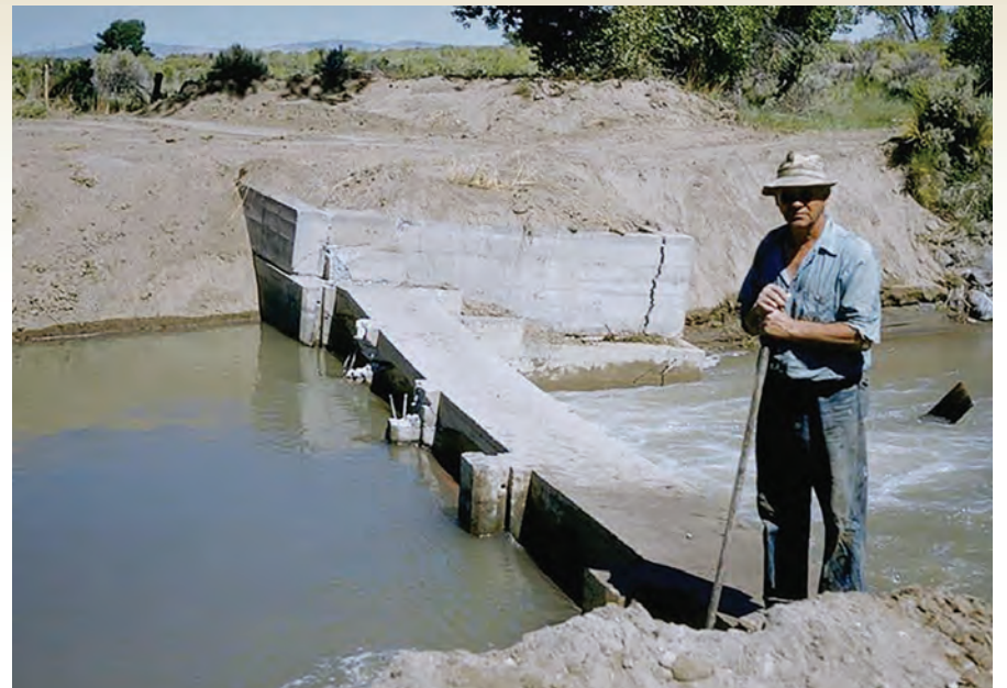
Coleman Dam on the Carson River was damaged so badly in the 1954 earthquake that it had to be completely replaced. Cal Berkley Library via Ernie Schank.
