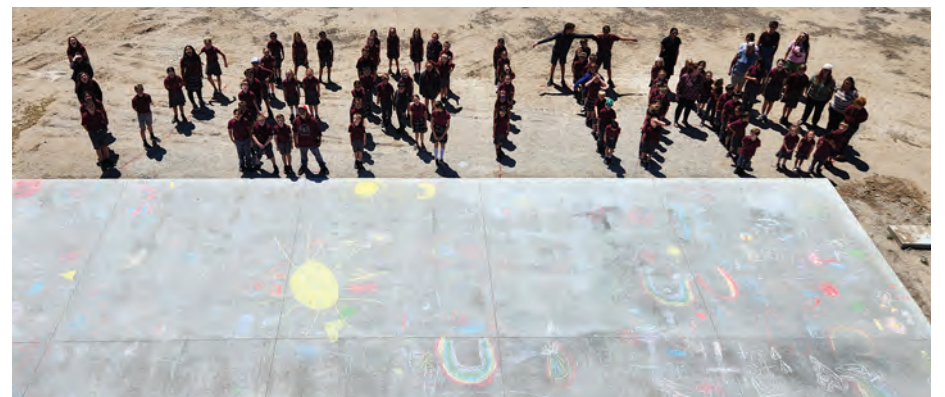
The students spell out “Veritas” on the newly poured foundation during last week’s groundbreaking celebration.
